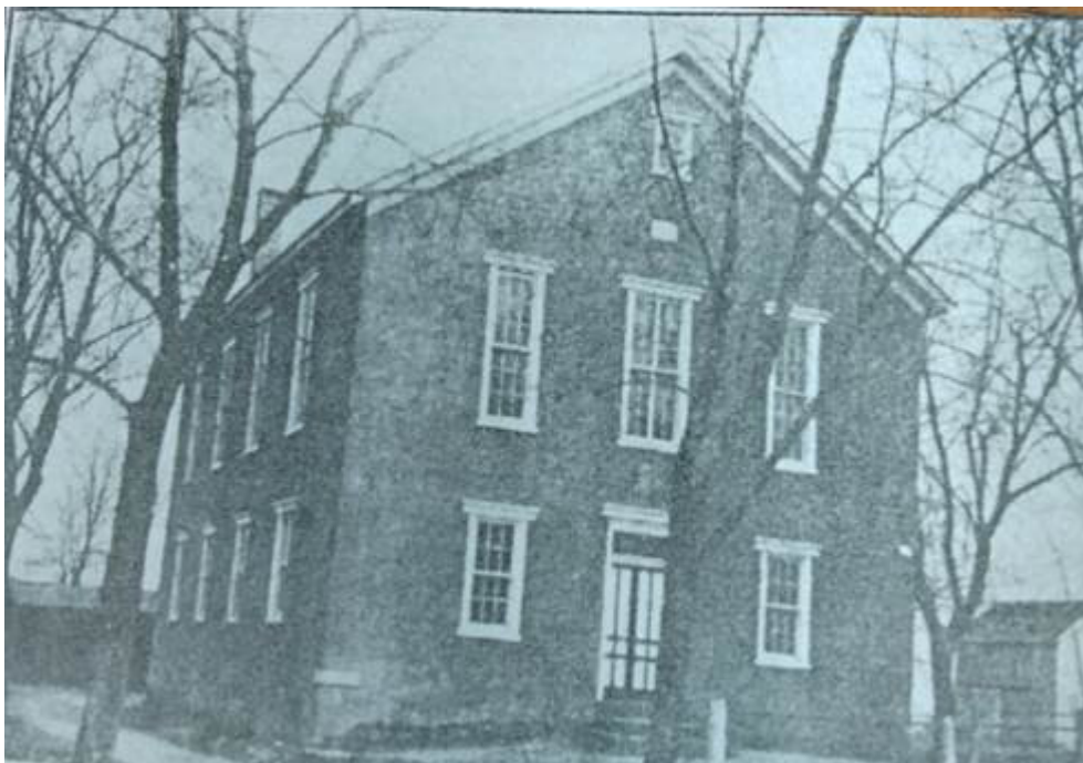
St. James Methodist Episcopal Church – Foundation Laid in September, 1873 (Later renamed Cedarville United Methodist Church)
